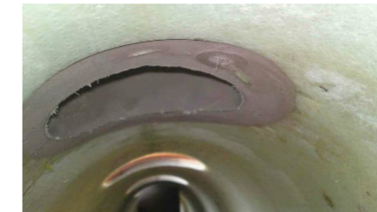
Grouted nozzle with mortar
