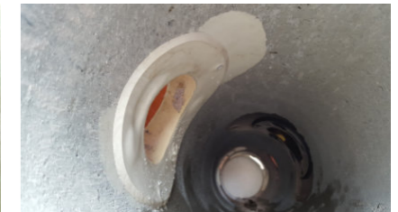
Grouted nozzle with epoxy resin
