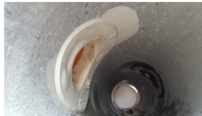
Grouted nozzle with epoxy resin
