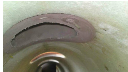
Grouted nozzle with mortar
